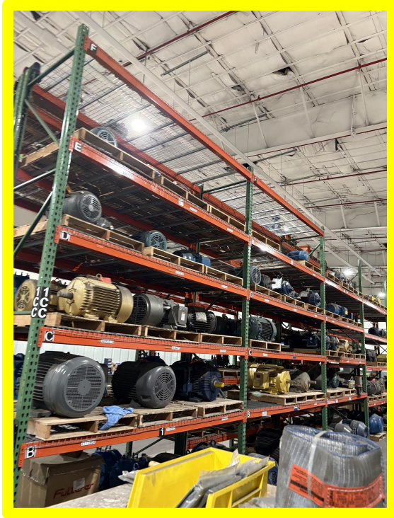
Ensure 18" minimum clearance between top of palletized load and sprinkler deflectors (NFPA 13) 7
