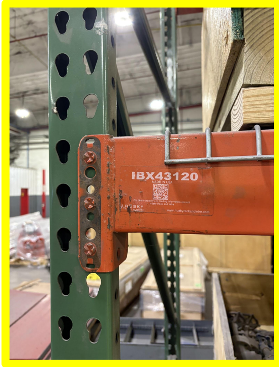
Missing Safety Clips 5
