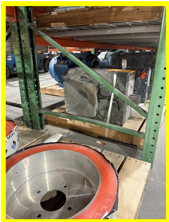
Row 1CB, Bay 5 Damaged Horizontal Brace 2
