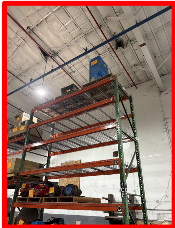
Ensure 18" minimum clearance. Loads should be distributed evenly across the full depth and width of the beam pair 6
