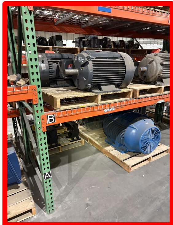
1CC, Bay 4 Damaged Beam 3
