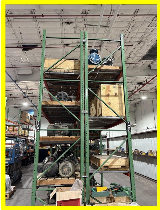
Rows 1CC & 1CB Longitudinal flue space less than 3" minimum between rows (NFPA 13) 8
